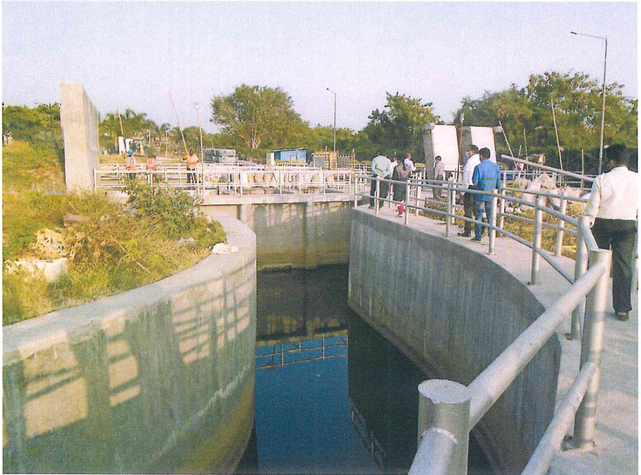
View of newly constructed I&D structure at Kukatpally Nallah.
