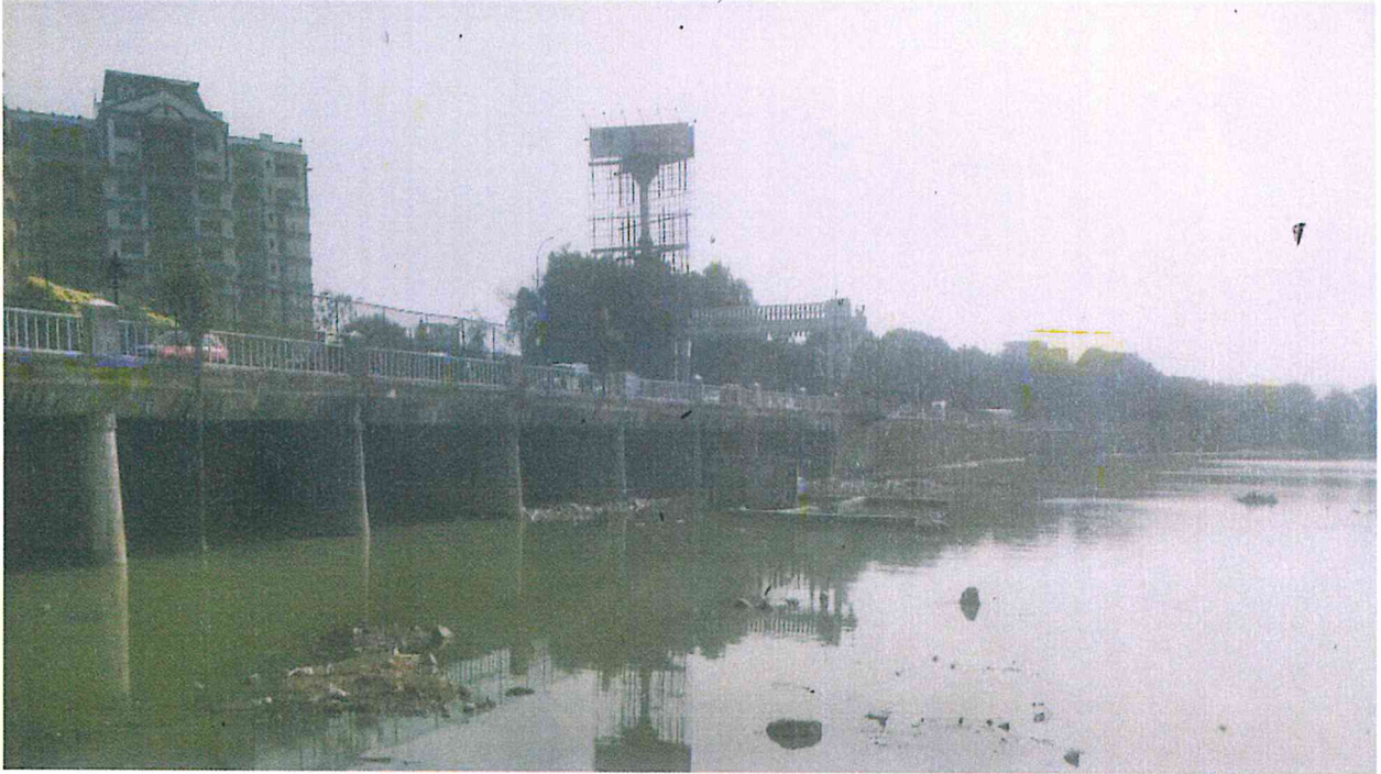
Photograph of the sluice gate no. 1
